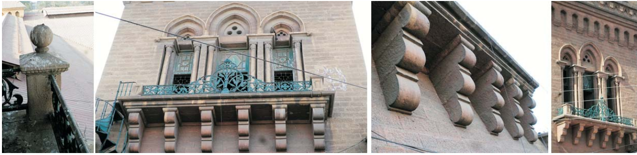
Figure 15: Images showing balcony, brackets under the balcony platform and pommel on top of the pedestal.
